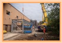
We also co-ordinated the complex arrangements and documentation required to utilise a specialist 160 ton crane for the removal of M&E across the external Roof area.
